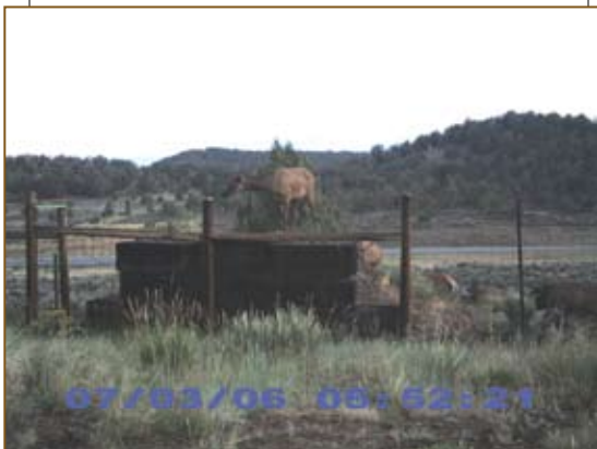
AN ELK USING AN ESCAPE RAMP ON US 550 NEAR RIDGWAY, COLORADO.
